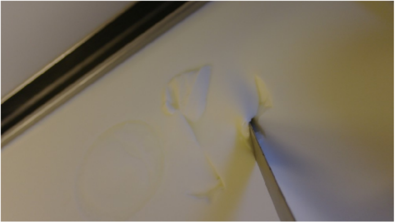
Checking for a clean break
